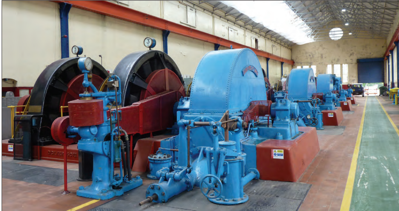
Historic hydro turbines once used to power the mighty Kinlochleven aluminium smelter, now preserved in the listed Turbine House and replaced by a bank of modern turbines churning out highly lucrative green power to the grid.
